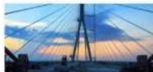
Wangdong Changjiang Bridge Anhui Province
